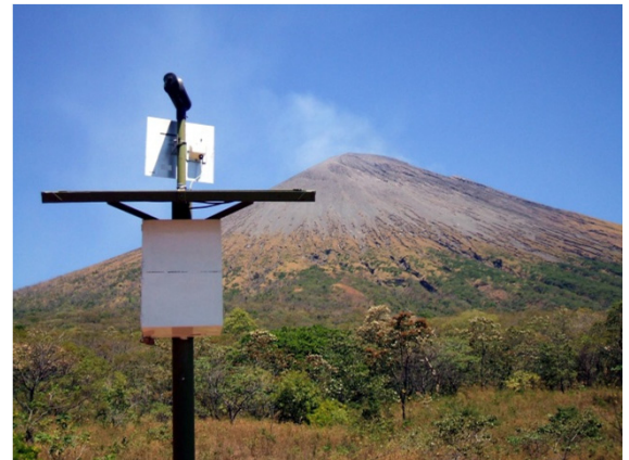
Solar Powered Remote Monitoring Station Volcán San Cristóbal, Nicaragua
